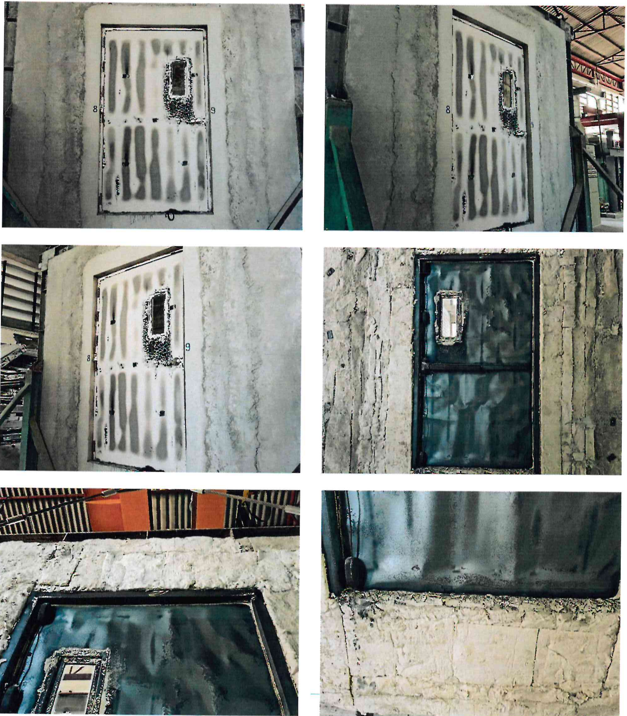
Figure D-3: The specimen after the test
